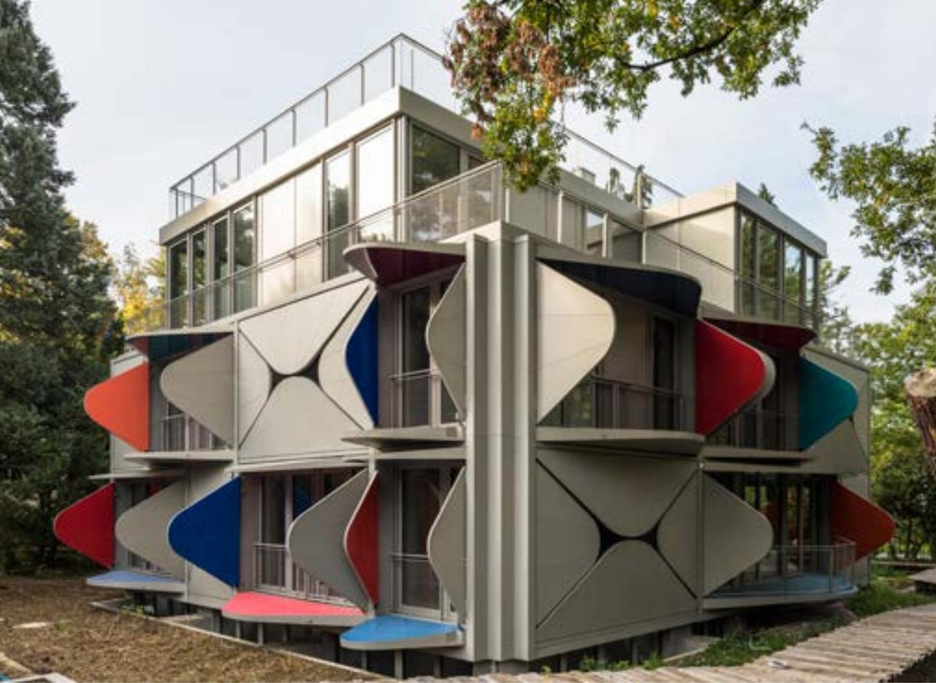
From left: the Ballet Mécanique apartment block in Zürich has panels that unfold to become balconies or sun louvers; when they are closed the building looks more like an art installation. The D\*Haus, scheduled to be built in Devon, is described as “the world’s first prefabricated
