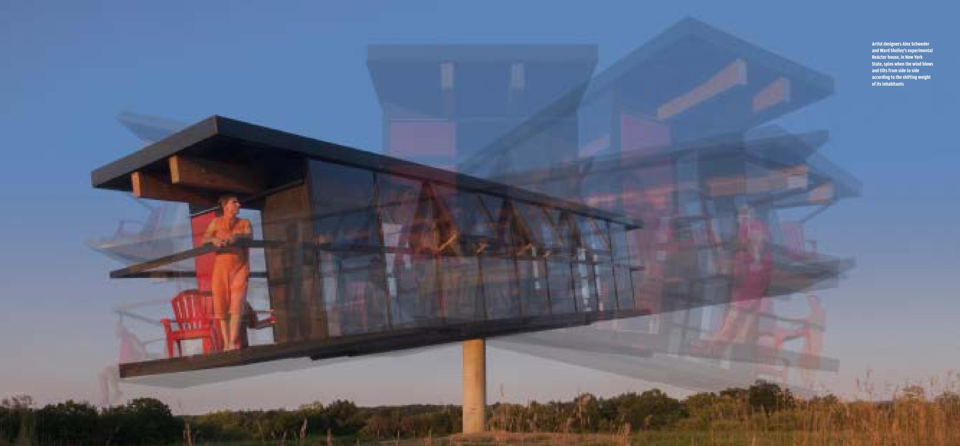
Artist designers Alex Schweder and Ward Shelley's experimental ReActor house, in New York State, spins when the wind blows and tilts from side to side according to the shifting weight of its inhabitants
